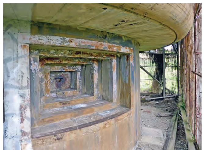
Fort Furggels: This close-defence bunker is encased in a substantial pitched roof structure which convincingly resembles a barn
